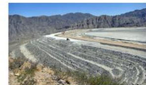
Figure 5. Modified centerline raise of a tailings storage facility (© Jon Engels)
